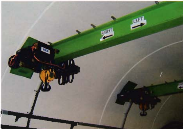
An Installation of two identical hoists inside the tunnel
